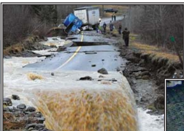
Flood damage in New Brunswick.
